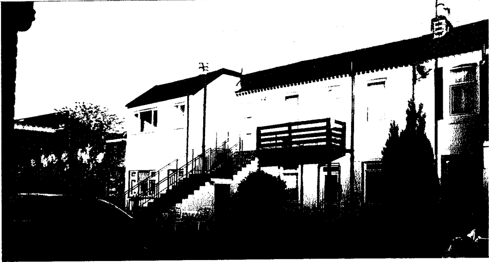
Two-storey housing dating from early – mid nineteenth century ↓
