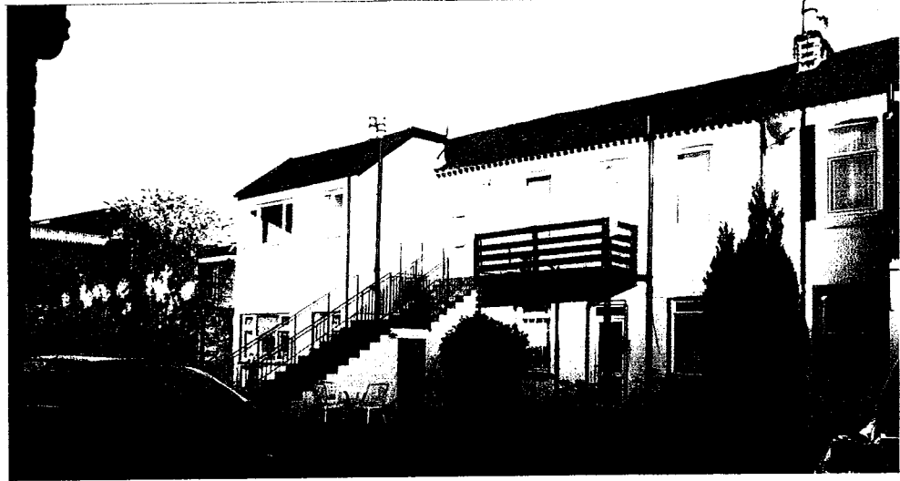
Two-storey housing dating from early – mid nineteenth century ↓
